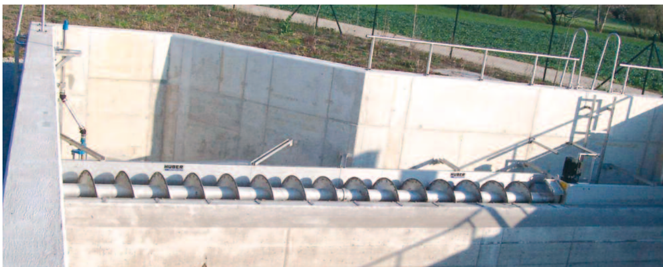
HUBER Storm Screen ROTAMAT® RoK1 for overflow screening at the WWTP inlet
