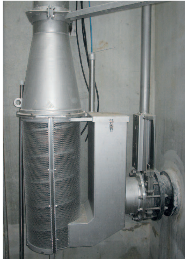
HUBER Pumping Stations Screen ROTAMAT® RoK4 screen flanged directly onto the incoming sewer to protect downstream pumps against coarse material
