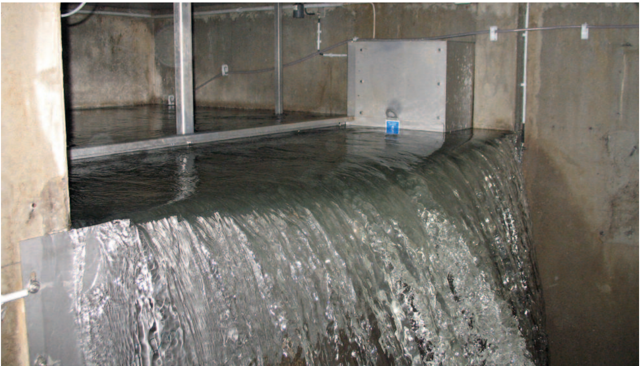
HUBER Storm Screen ROTAMAT® RoK2 with discharge flow measurement during storm events
