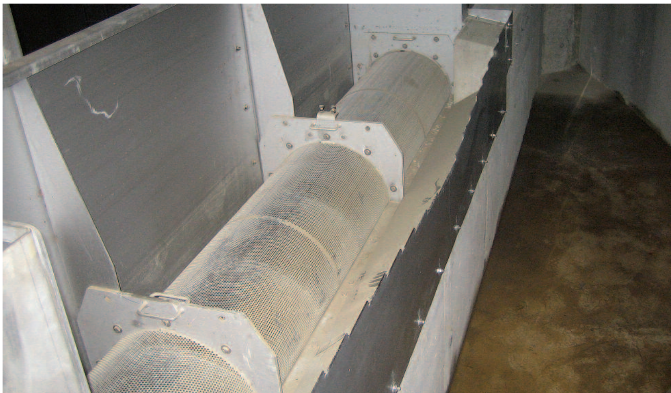
Stormwater screening combined with overflow measurement: HUBER Storm Screen ROTAMAT® RoK2 with gauging weir
