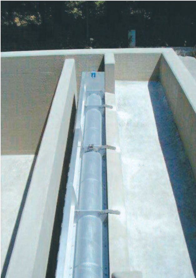
HUBER Storm Screen ROTAMAT® RoK2 installed at the overflow of a stormwater retention tank
