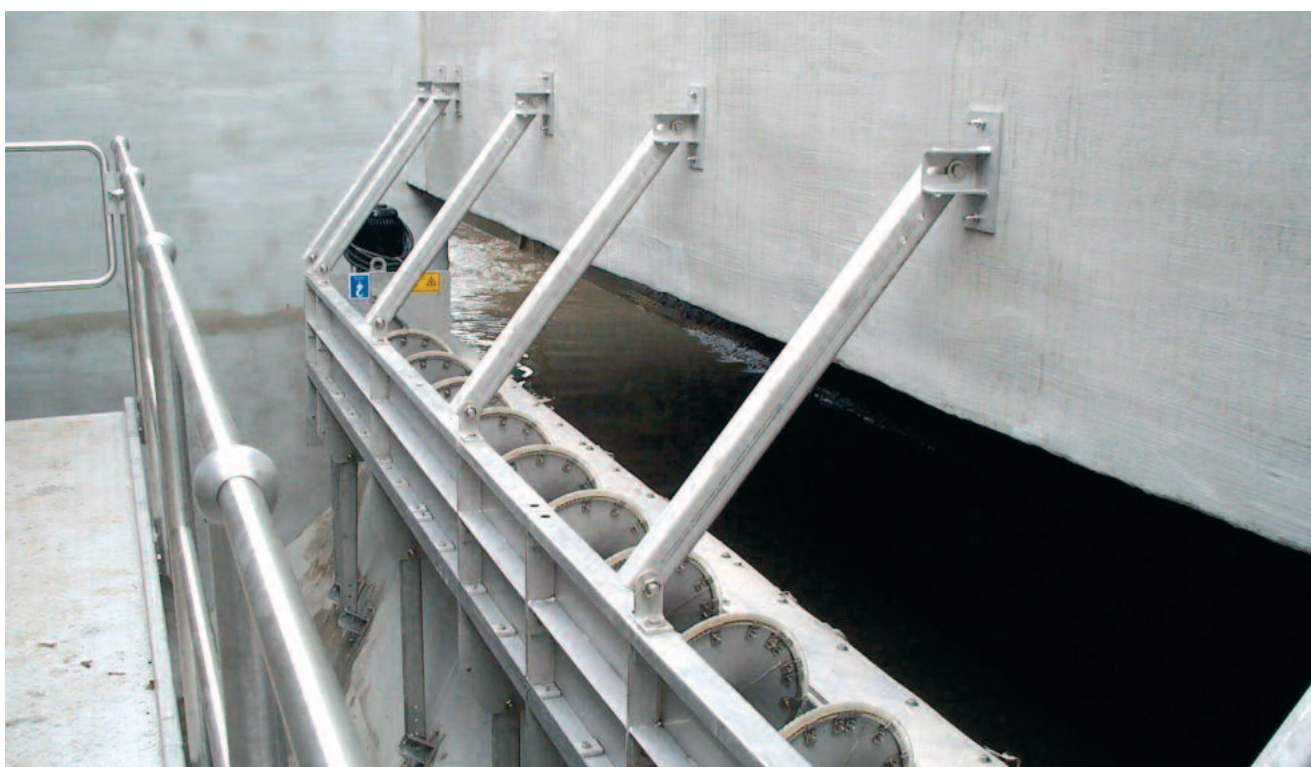
HUBER Storm Screen ROTAMAT® RoK1 installed at a stormwater overflow tank
