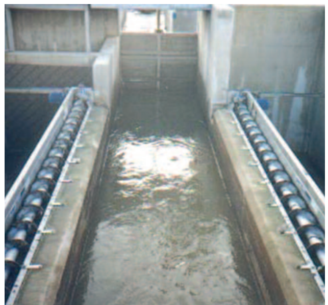
HUBER Storm Screen ROTAMAT® RoK1 units installed on both sides of the WWTP inlet for increased throughput
