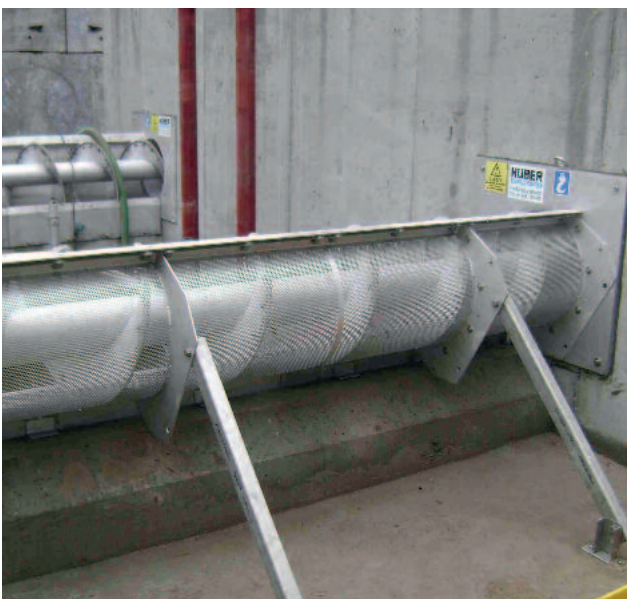
HUBER Storm Screen ROTAMAT® RoK1 installed at an angle of 60° to save horizontal space
