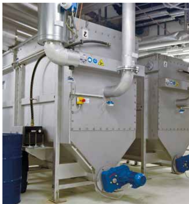
Municipal wastewater; 2x RoWin size 8; heat extraction capacity 560 kW heating / 1,000 kW cooling.
